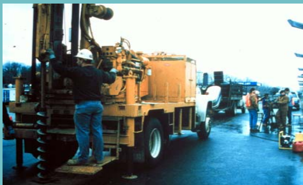
Steam cleaned core barrels advanced thru steam cleaned, hollow stem augers
